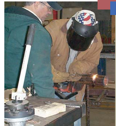
A pipefitter cuts steel pipe with a cutting torch.
